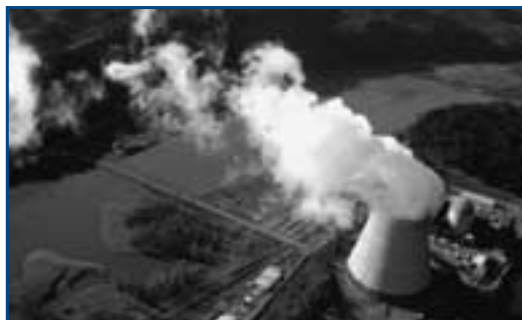
Figure 22. Nuclear power plant
