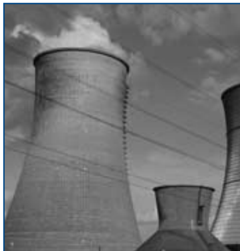
Figure 16. Nuclear Power Plant
